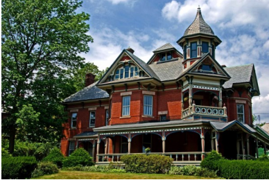
1093 Dwight Street Holyoke 1886 totally restored
