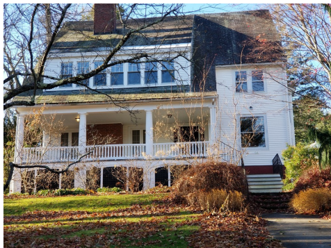
94 Crescent St Northampton 1910 under- going a total restoration
